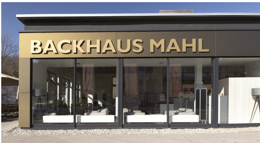
FIG. 5.8. Point fixing system through the cladding, with mullions. Backhaus Mahl, Albstadt-Tailfingen – Germany (Source: © Courtesy of Alucobond, © Elisabeth Leblanc)
