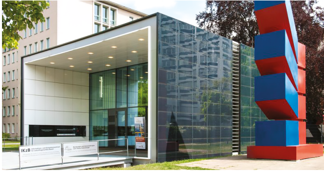
FIG. 1.9. Photo of the building of the Project Efficiency House Plus with E-mobility in Berlin (Source: photo from https://www.solarwende-berlin.de/allgemein/masterplan-solarcity-berlin/wettbewerb-architektur Free License)
