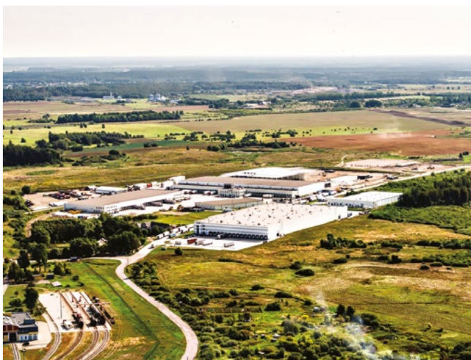
FIG. 8.2. Picture BLC logistics center (Source: own elaboration, 2019)
