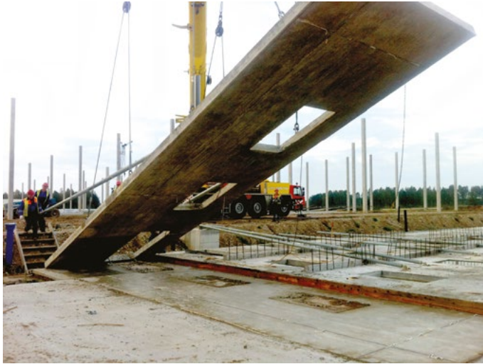
FIG. 8.2. Tilt-up panel (Source: own elaboration, 2018)
