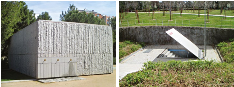
FIG. 4.10. Madrid-Rio Project, small objects located in the new public space, in Madrid, Spain. Left: Infrastructure and fountains with granite stone. Right: Emergency exit from underground tunnel (Source: photos by M a A. Flórez de la Colina, 2019)
