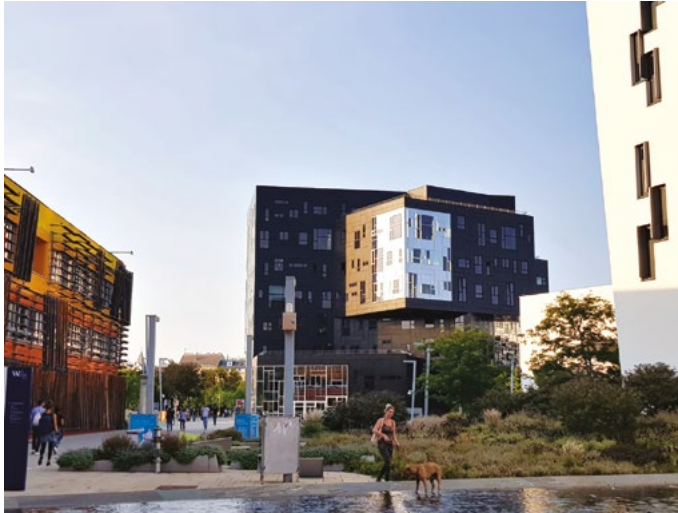
FIG. 4.3. University area in Vienna – Austria (Source: photos by A. Vidales, 2020)
