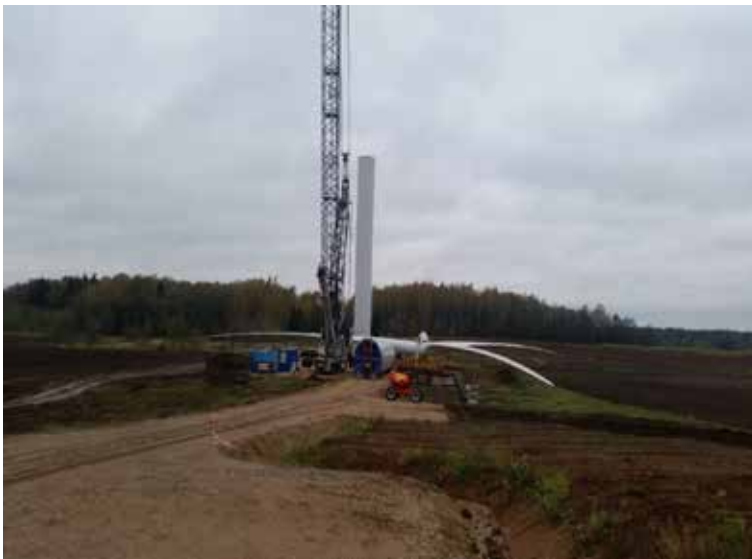
Fig. 3.13. Installation of wind turbine elements in a field (Source: photo by K. Jasiūnas)
