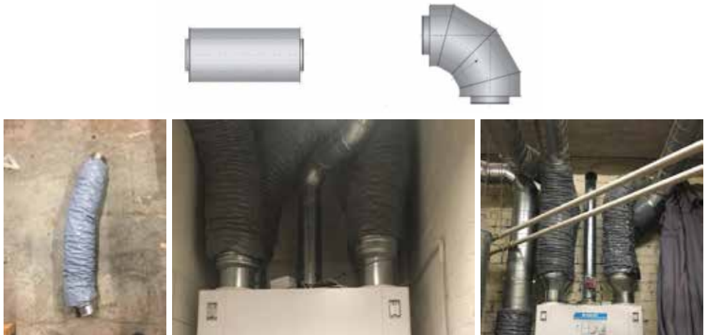
Fig. 8.15. Noise silencer types (Source: Bilinskienė, 2017; R. Bilinskienė's private archive; WEB-1)
