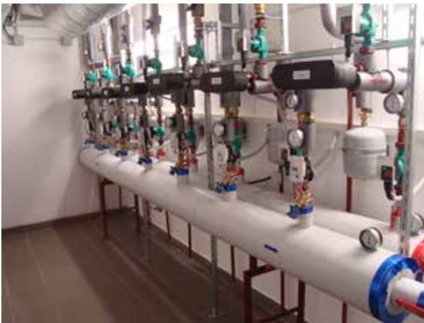
Fig. 7.19. Circulation pumps in a boiler room (Source: photos by T.J. Teleszewski)
