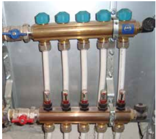
Fig. 7.4. The connection of the central heating installation: A) pipes distributed in a two-pipe loop B) the radiant heat manifolds (Source: T.J. Teleszewski's private archive)
