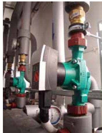
Fig. 7.19. Circulation pumps in a boiler room (Source: photos by T.J. Teleszewski)
