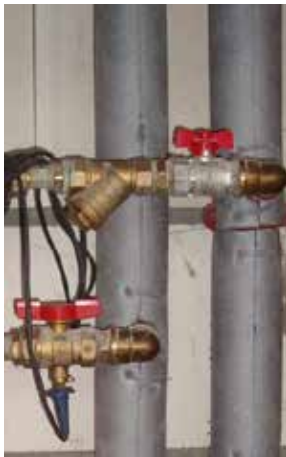
Fig. 7.4. The connection of the central heating installation: A) pipes distributed in a two-pipe loop B) the radiant heat manifolds (Source: T.J. Teleszewski's private archive)
