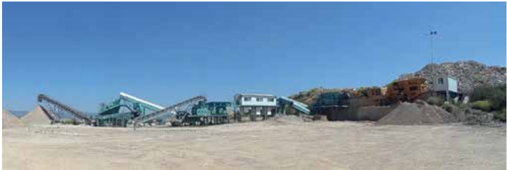
Fig. 3.21. Elements of a recycling plant. GECORSA, Córdoba, Spain (Source: J. R. Jimenez's private archive)
