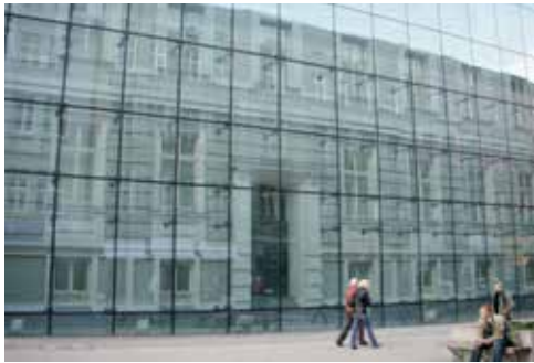
Fig. 1.28. Inbuilt in the new building, the elevation of a 19th century tenement house with a built over glass facade – Old Brewery Shopping And Art Centre (Poznań, Poland) (Source: photos by M. Kłopotowski.)
