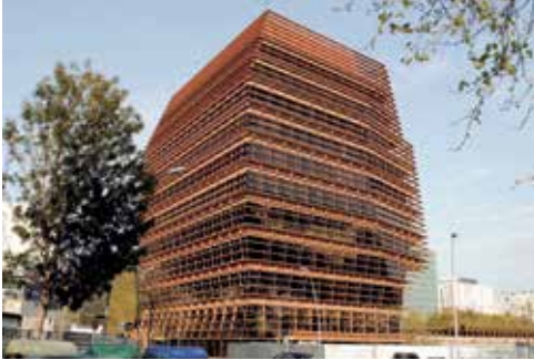
Fig. 1.11. Windows protected from excessive sun and light. A) Brise-soleils on elevations of Edifici CMT 22 @ (Barcelona, Spain), B) Automatically regulated translucence facade of Institut du Monde Arabe (Paris, France) (Source: photos by M. Kłopotowski)
