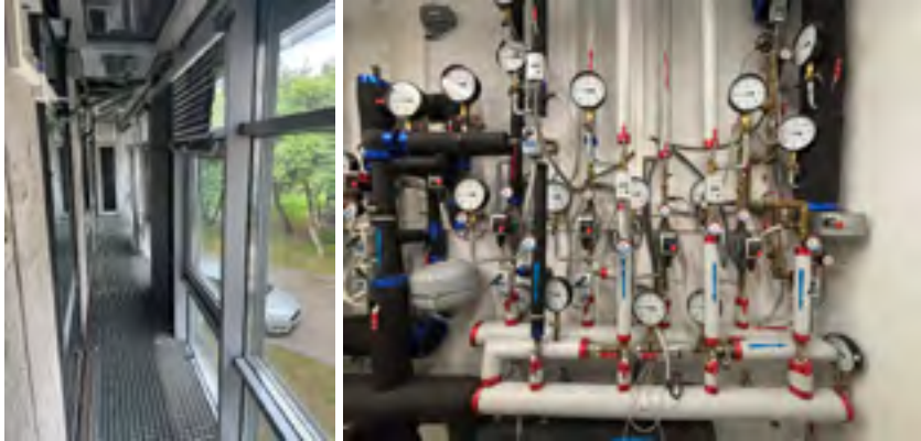
Photo 2.2. Double glass facade with TABS hot air distribution equipment visible; heating and cooling circuits with automation equipment – actuators, adjustable circulation pumps and heat meters. Photo: M. Tur 2025.
