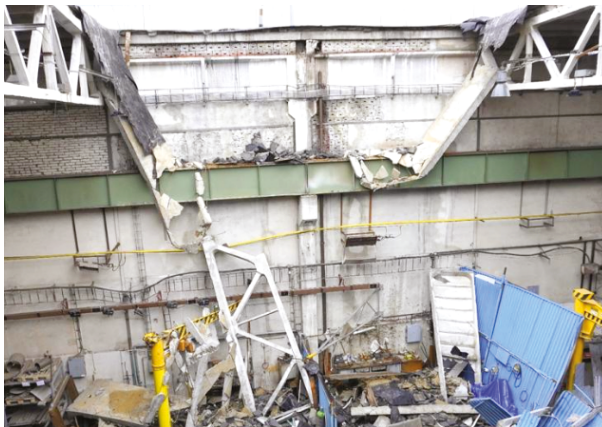
FIG. 1. Truss girder collapse in the Czech Republic from 2023 [1]
