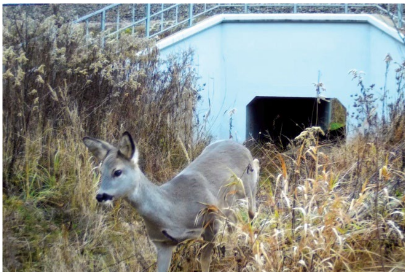
Figure 3. Animal crossing under the railway line E-75 Rail Baltica “Warsaw–Białystok–Lithuania” border as a habitat connectivity measure implemented during the upgrade co-financed by the CEF
