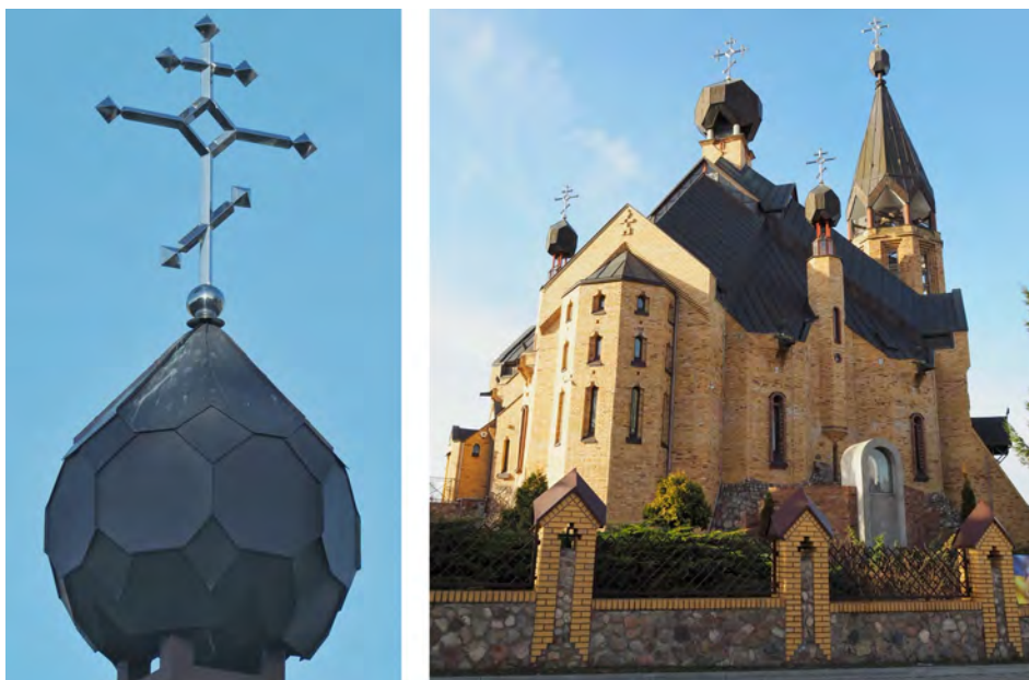
Figure 2.18: Orthodox Church of the Resurrection in Białystok, designed by Jerzy Uścińowicz, 1991 – 1994. Shape of dome fragment resembling flat 8 - 4 - 8 semi-formal tessellation (dome from left), shape of other domes resembling fragment of Archimedean tetrahedron (Fig. 2.16) – square bordered by four regular hexagons (four domes from right), photo by M. Koźniewski
