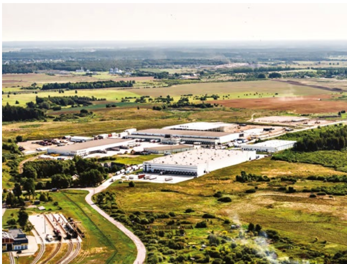
FIG. 8.2. Picture BLC logistics center (Source: own elaboration, 2019)
