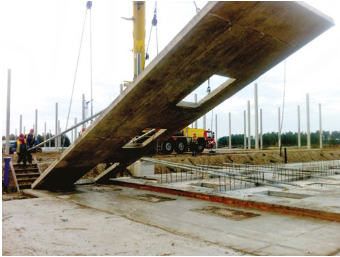
FIG. 8.2. Tilt-up panel (Source: own elaboration, 2018)
