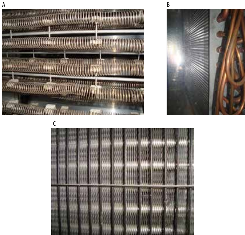
Fig. 8.17. Elements of the air heating section: A) coiled heating elements for an electric heater, B-C) hot water coils (Source: T.J. Teleszewski's private archive)
