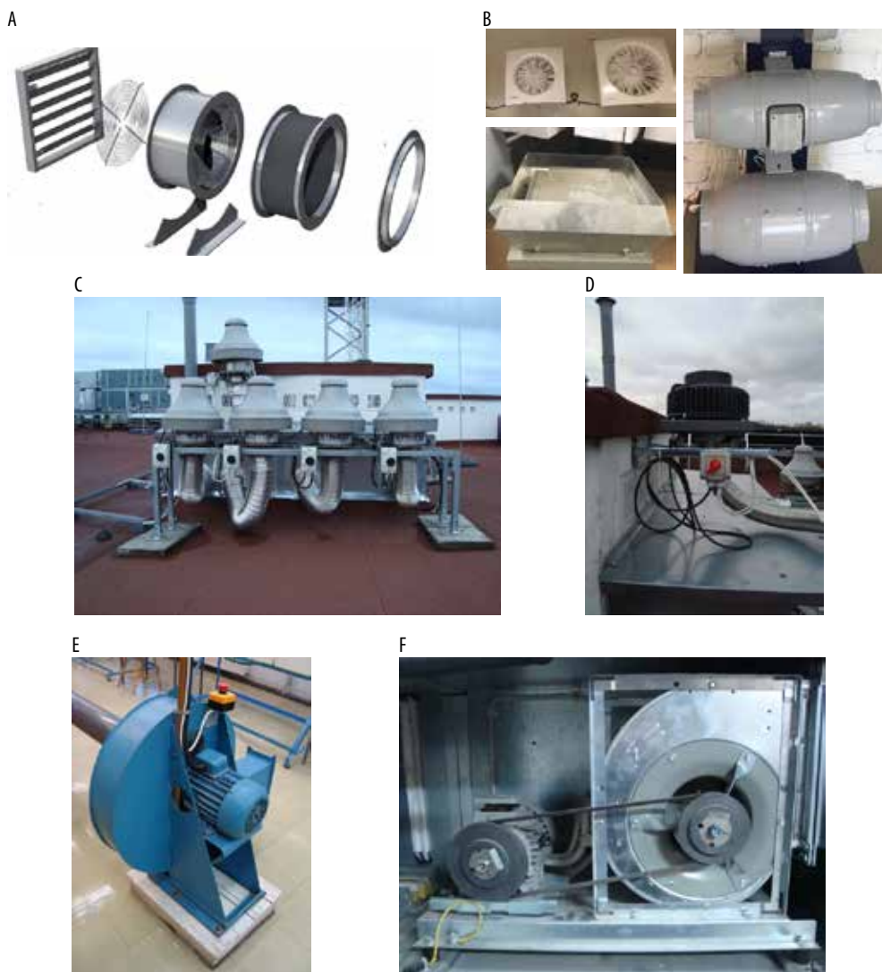
Fig. 8.7. Examples of fan constructions: A), B) an axial fan for installation in the ventilation duct and on the roof, C), D) axial fans installed on the roof, E) a centrifugal fan, F) a cross flow fan installed in the AHU unit (Source: Bilinski  n  , 2017; WEB-1; R. Bilinski  n  's private archive; photos by T.J. Teleszewski)
