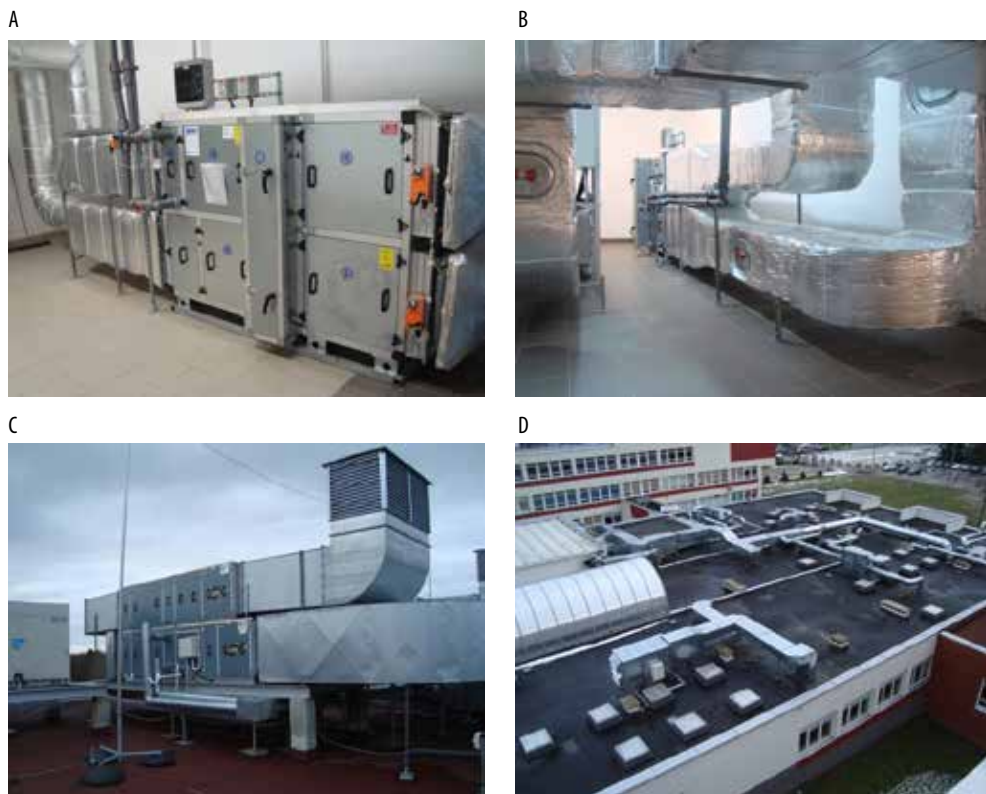
Fig. 8.5. Location of the AHU: A-B) in the basement, C-D) on the roof (Source: photos by T.J. Teleszewski)
