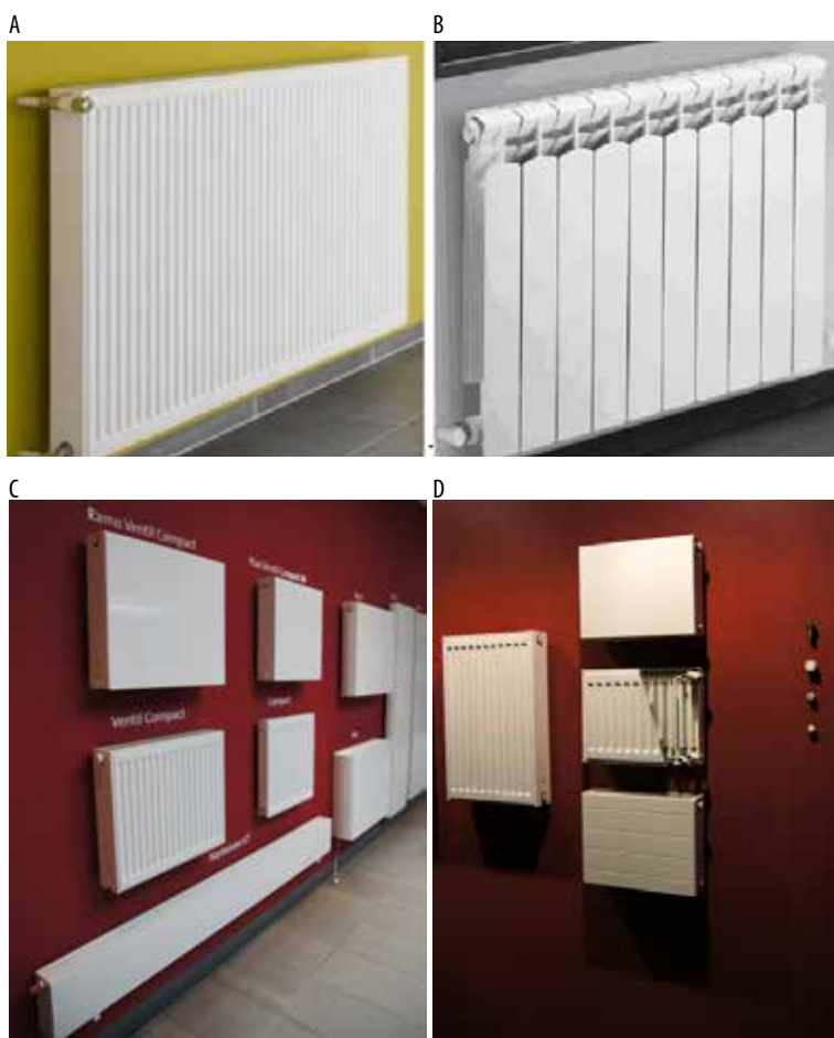
Fig. 7.5. Examples of heating devices. Radiators: A) panel radiator, B) column cast iron radiator C-D) different surfaces of panel radiators (Source: A) Bilinskienė et al., 2012, B) Bilinskienė, 2017, C) photo by D.A. Krawczyk, D) photo by E. Szatyłowicz)
