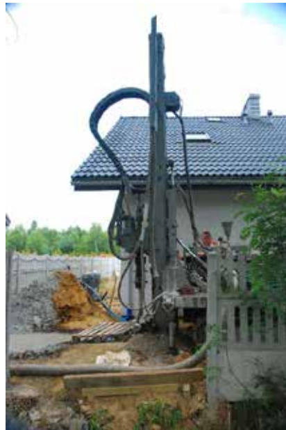
Fig. 5.24. Drilling of boreholes (Source: Smuczyńska, 2015)
