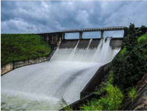
Fig. 1.13. Photo of Hydropower Plant (Source: WEB-1)
