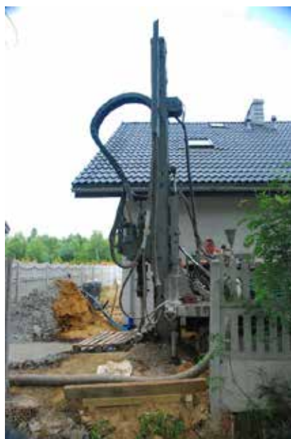
Fig. 5.24. Drilling of boreholes (Source: Smuczyńska, 2015)
