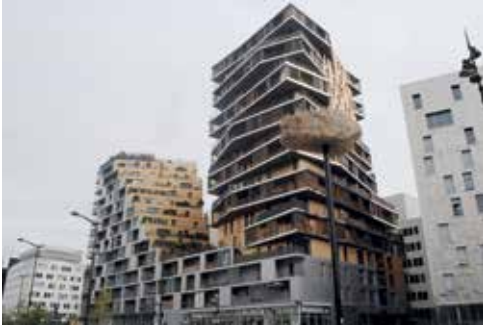
Fig. 2.22. Balconies surrounding a building completely change its spatial reception – Bâtiment Home in Paris XIII, France (2012-2015, architect Hamonic + Masson & Associés) (Source: photos by M. Kłopotowski)
