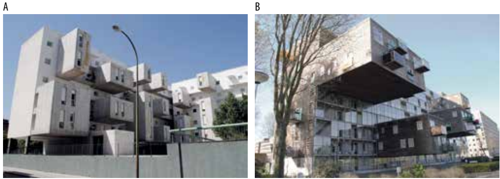
Fig. 2.30. Residential buildings with rooms and flats in large cantilever constructions. A) 102 outthrust social dwellings in a block of flats in Carabanchel, Madrid, Spain (2008, architects Ignacio Borrego, Néstor Montenegro and Lina Toro – Dosmasuno Arquitectos), B) The WoZoCo in Amsterdam, Netherlands (1994-1997, architects MVRDV) (Source: photos by M. Kłopotowski)
