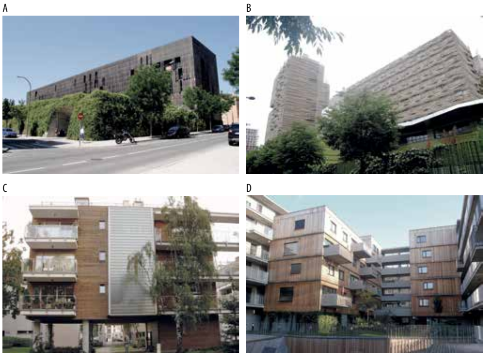
Fig. 2.33. Wood as a “new” pro-ecological building material. A) Moving shutters over the balconies around the Carabanchel Social Housing, Madrid, Spain (2007, architects Farshid Moussavi and Alejandro Zaera-Polo – Foreign Office Architects), B) Wooden openwork elevations School Group and Student Housing – Clichy –Batignolles, Paris, C) Wood-finished facades of the Allegretto Housing Complex in Eko Park in Warsaw, Poland (1999-2003, architects Stefan Kuryłowicz, Paweł Gumuła, Maria Saloni-Sadowska), D) Wood-finished facades and floors in Holzwohnbau in Seestadt Aspern, Vienna, Austria (2011-2015, architects Alfred Berger, Tiina Parkkinen – Architekten Berger + Parkkinen Ziviltechniker GmbH) (Source: photos by M. Kłopotowski)
