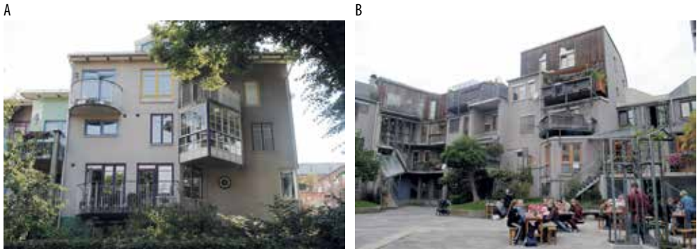
Fig. 2.15. Multi-family houses realized as a result of the process of social participation consisting in the cooperation of an architect with a particular user. A) A Bo 100 building in Malmö, Sweden (1987-1991, architect Ivo Waldhör with the team), B) Wohnbau Alte Poststraße (1982-1984, architects Michael Szyszkowitz and Karl Kowalski) (Source: photos by M. Kłopotowski)
