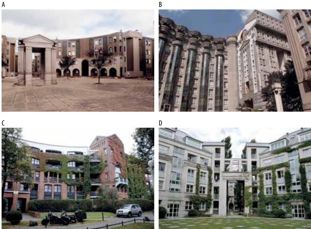
Fig. 2.14. Postmodernist realizations of housing development from the 1980s. A) Les Arcades du lac le Viaduc in Saint – Quentin-en-Yvelines, France (1982, architect Ricardo Bofill), B) Les Espaces de Abraxas in Noisy-le-Grand, France (1982, architect Ricardo Bofill) C) IBA Wohnanlage in Berlin, Germany (1985, architect Rob Krier), D) An apartment Development on the Tegel Waterfront in Berlin, Germany (1986-1986, Moore Ruble with the team) (Source: photos by M. Kłopotowski)
