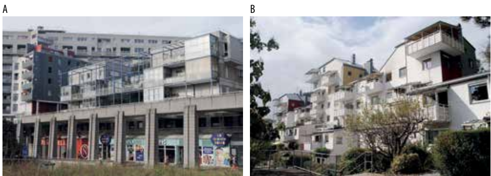
Fig. 2.16. Neomodernist housing developments from the 1980s. A) Social Housing at La Villette, Paris, France (1981-1997, architect Gérard Thureau), B) Wienerberger Gründe in Graz, Austria (1981-1997, architects Ralph Erskine and Hubert Rieß) (Source: photos by M. Kłopotowski)
