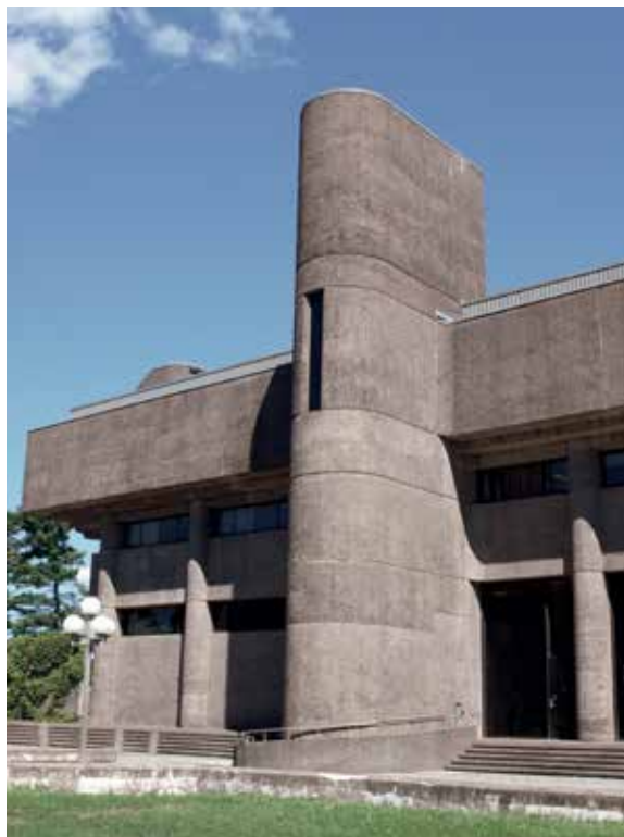
Fot. 94. Douglas Orr, service tower w Albert C. Jacobs Life Sciences Center – Trinity College w Hartford, 1965-1967; fot. autor
